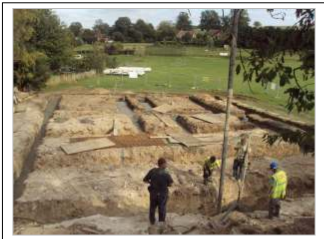
Progress! The footings are in! (c/o Ina Schmitz-Williams)
